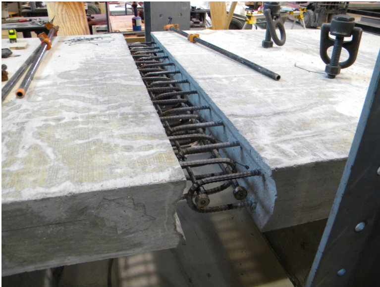
Longitudinal Joint Prior to Closure Pour
